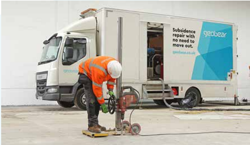
Figure 7: Stages of geopolymer injection
