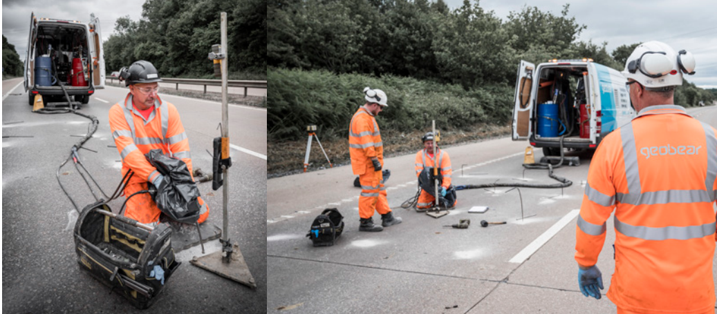
Photo 1: The drilling process at predetermined locations
