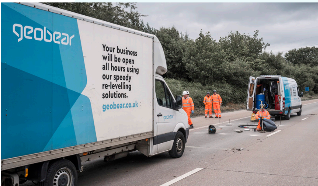
Photo 2: Geopolymer injection process
