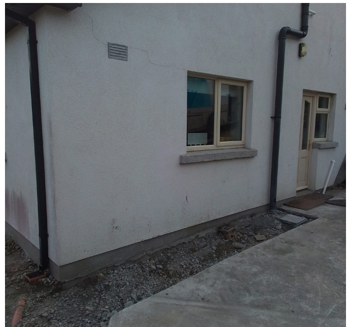
Post works, clean site
