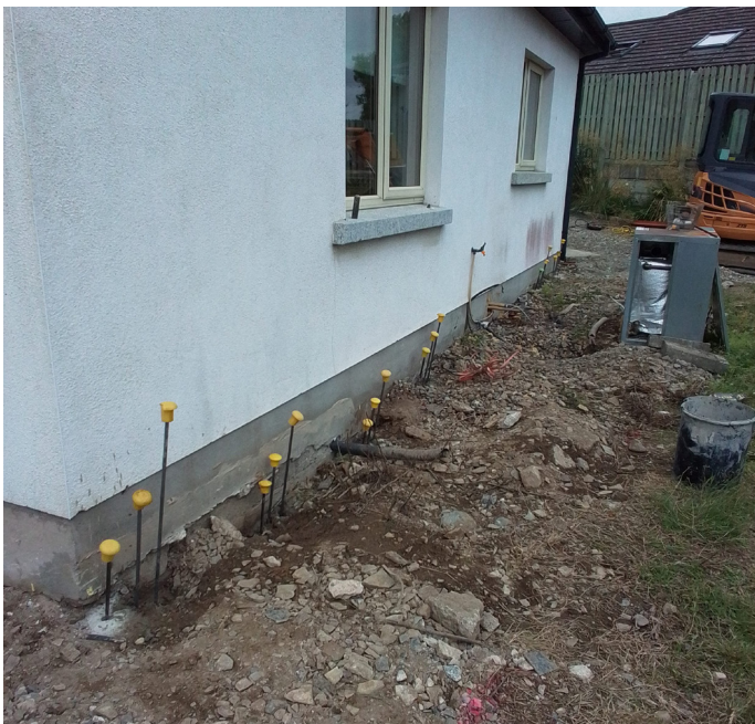
Work in progress, minimal intrusion
